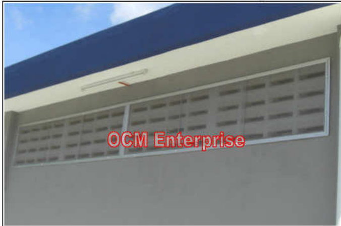
Composite (FRP) Louvers Window & Alu Netting TNB Sub Station Signage
